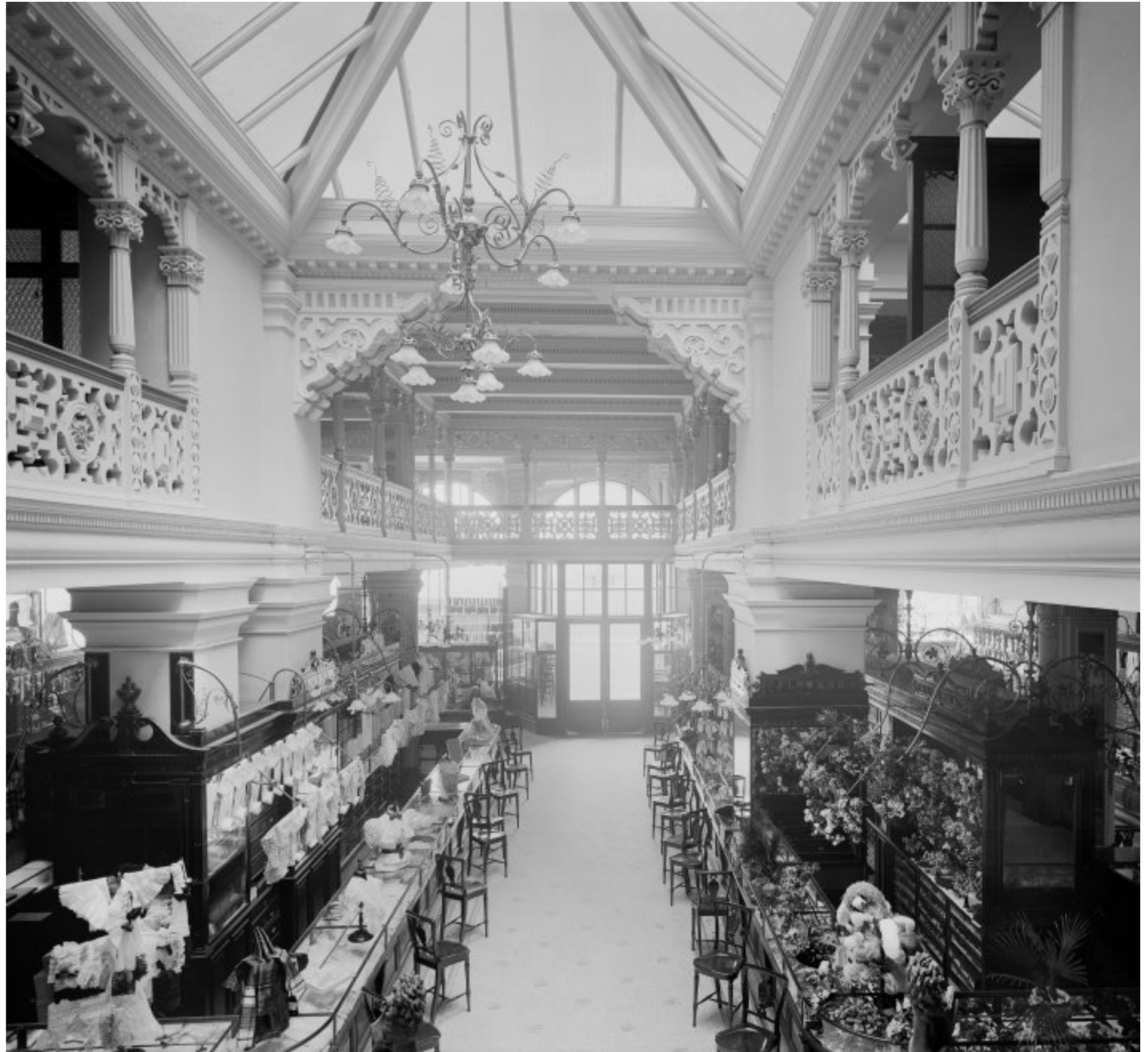
Mezzanine void and skylight which have both been lost by modern floorplate infills © Courtesy of HES (Bedford Lemere and Company Collection)
