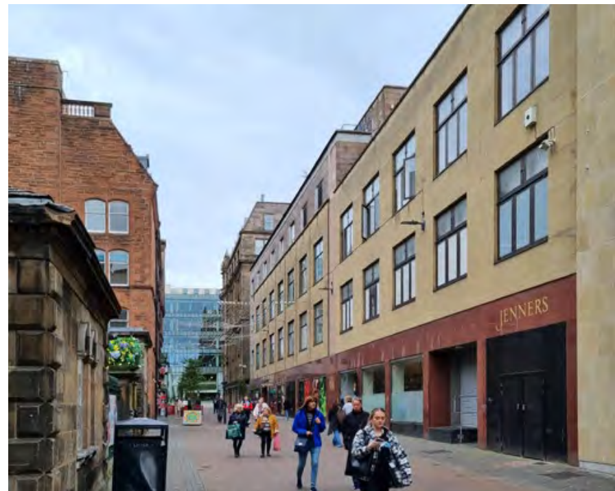
E - 1960's and 1970's building from Rose Street
