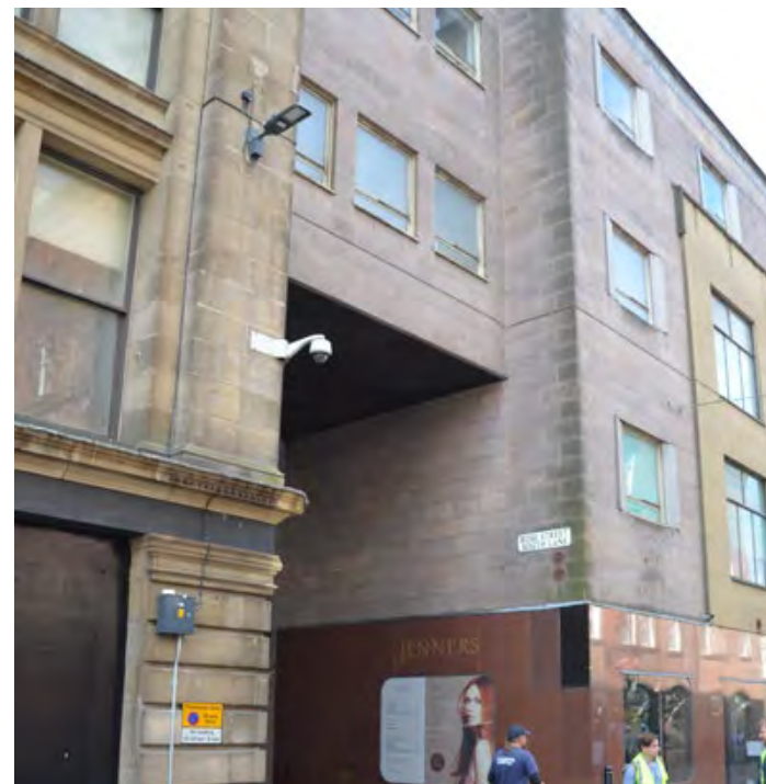
Doddington sandstone on Rose Street façade
