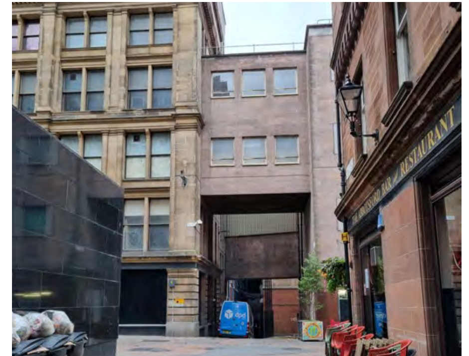
4 – Bridge link between 1905 extension and 1960's building
