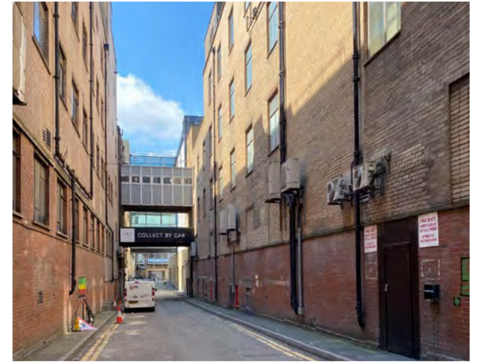
2 – Rose Street South Lane with bridges owned by Marks and Spencer
