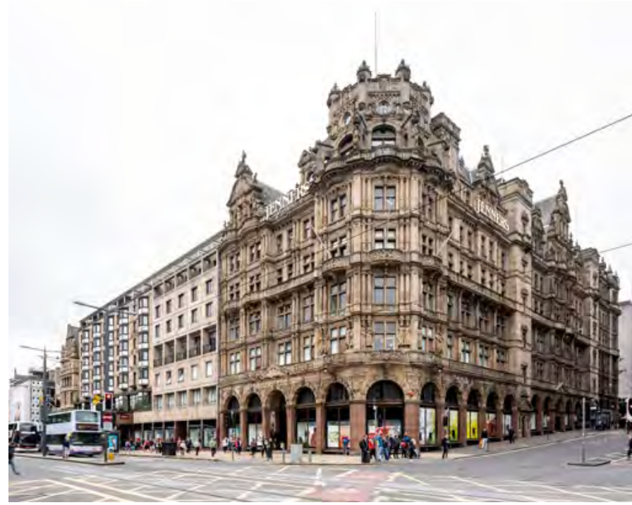
B - View from junction of Princes Street and South Saint David Street
