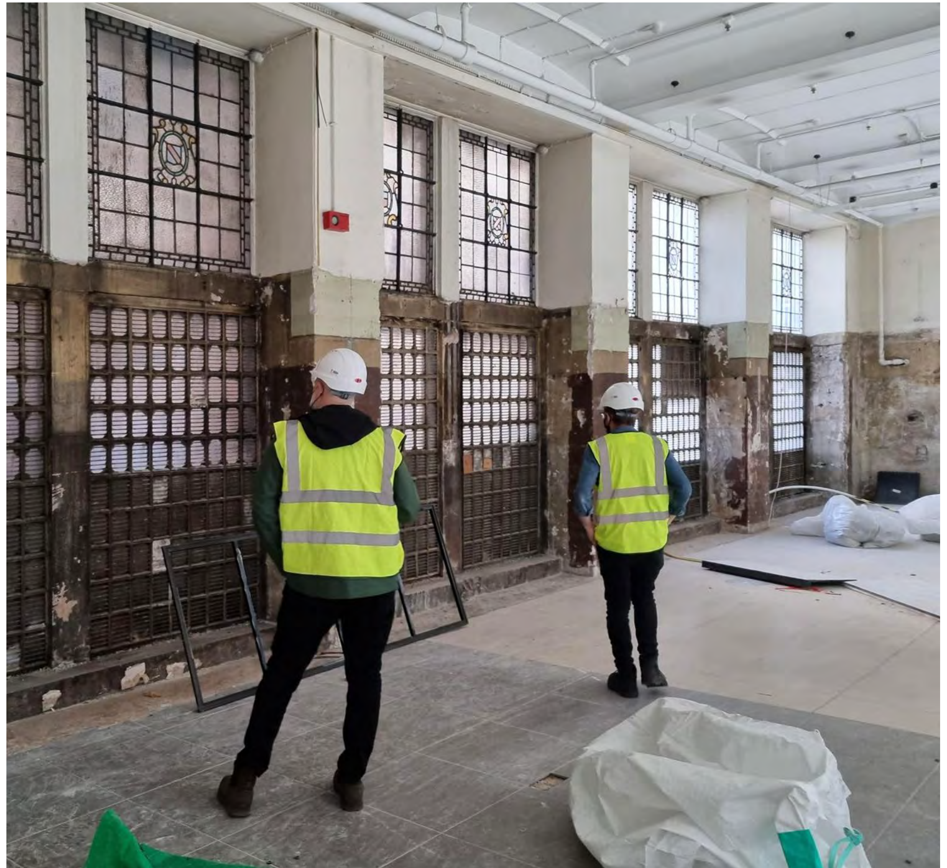
Opening up of historic windows during strip out works
