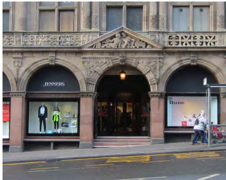
C - 1895 South St David Street entrance with 500mm level difference
