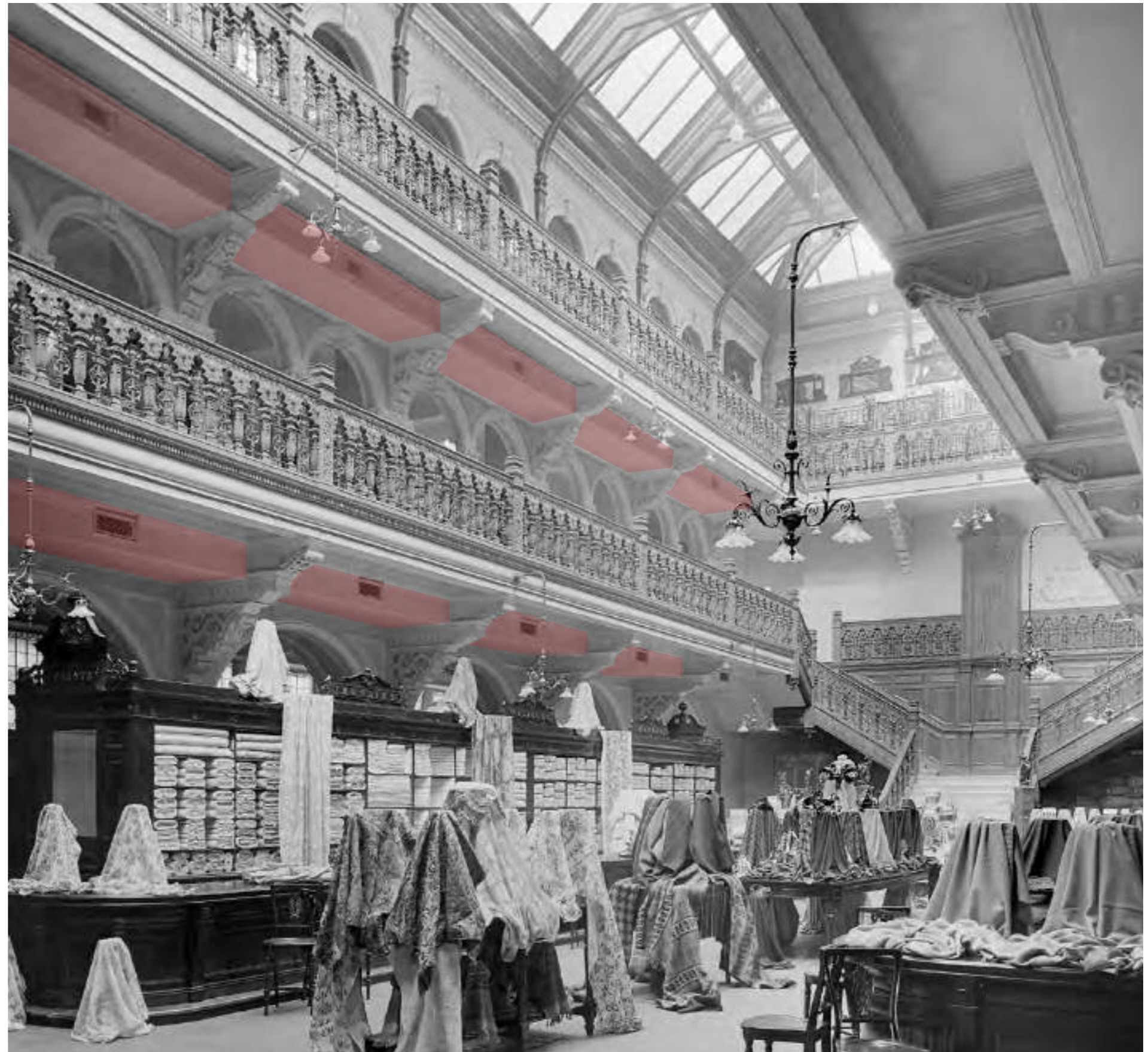
1905 photograph highlighting original air vents
