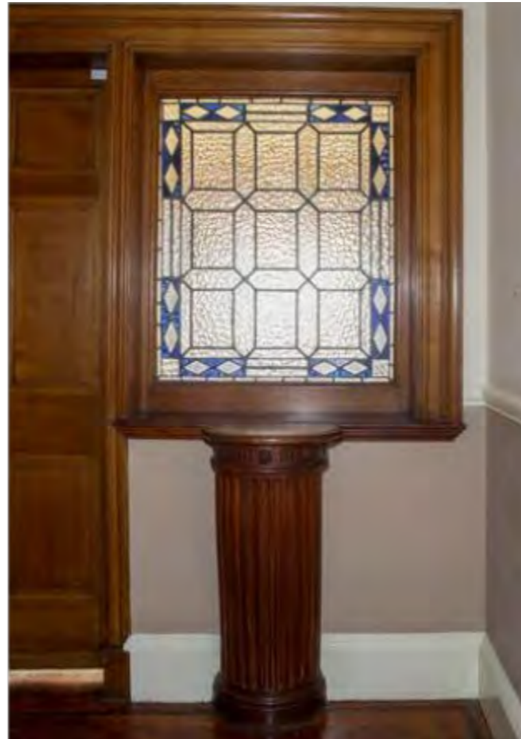
Historical timber lining in the former director's suite, 3F
