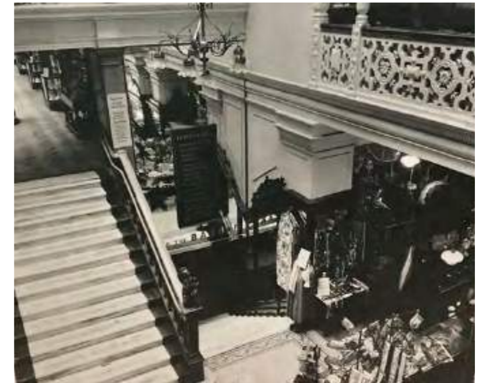
Collection of materials (timber parquet and balustrade, marble treads, ironwork)
