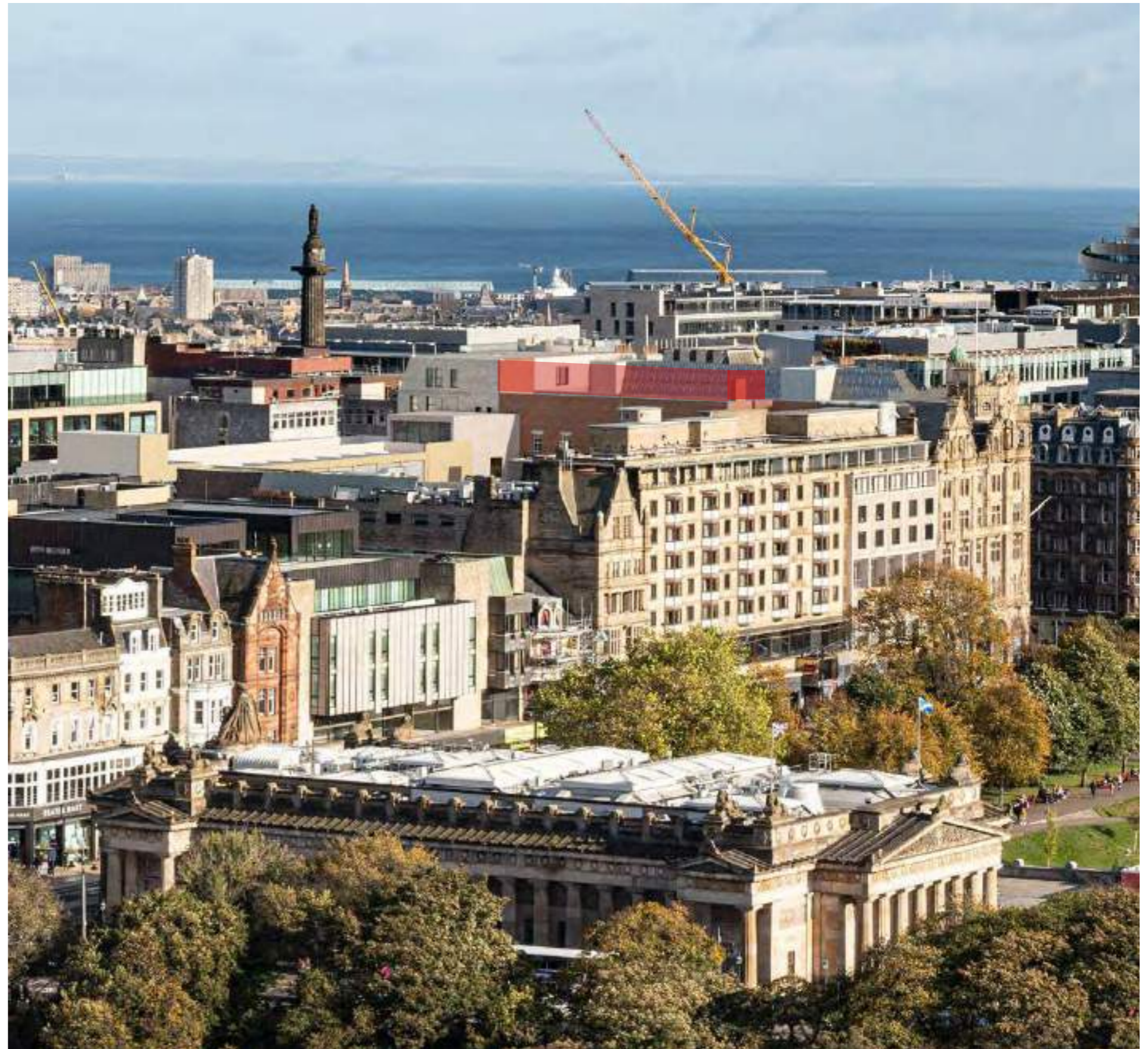
Proposed verified view from The Mound - red volume indicates original volume of west wing extension, subsequently reduced during pre-application discussions
