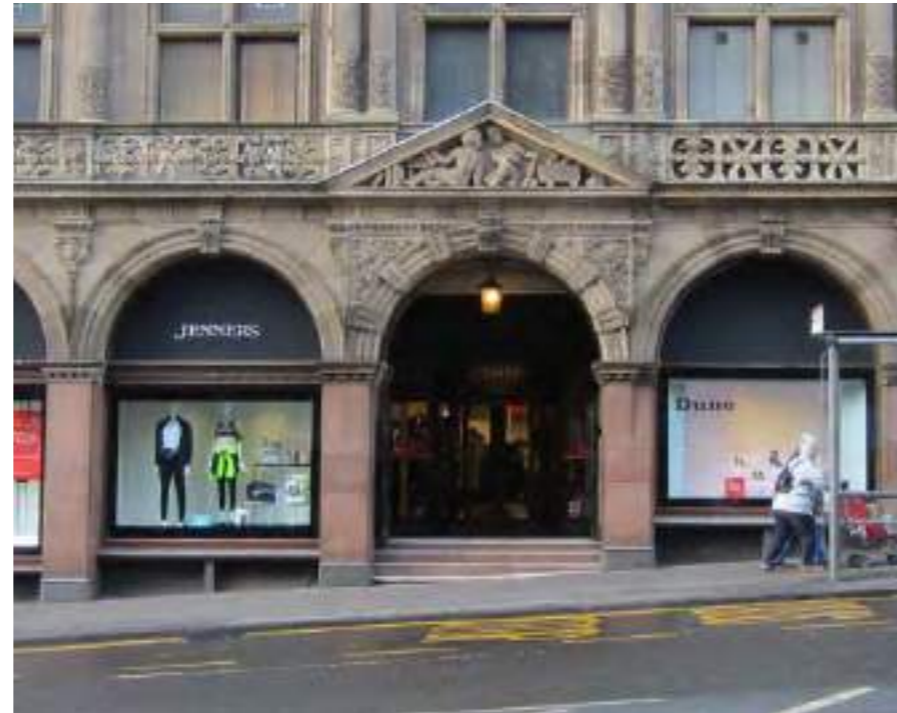
Existing 1895 South St Davids Street entrance
