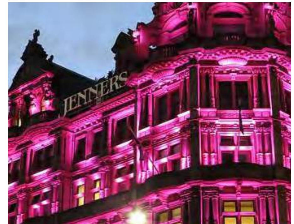
Colour changing façade lighting can be found in a few locations nearby, including the previous lighting scheme for The Jenners Building's Façade. Coloured light is not the most suitable way to render material qualities and emphasize stone finishes. A warm/neutral white light tends to be more sensible for historical façades and it is recommended for historical buildings.
