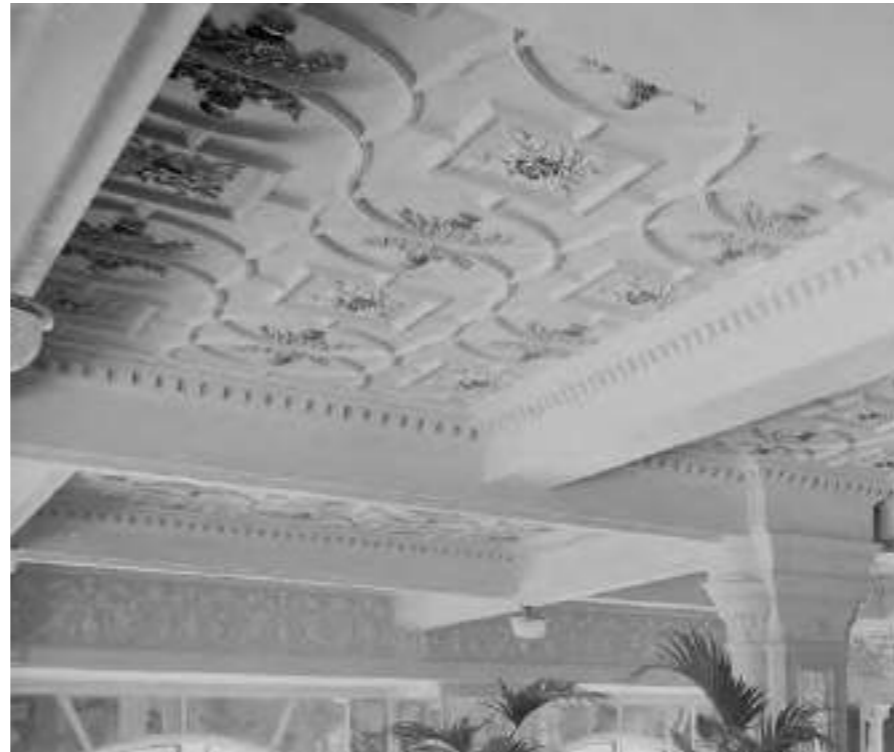
Historic mezzanine ceiling with painted decorative plasterwork
