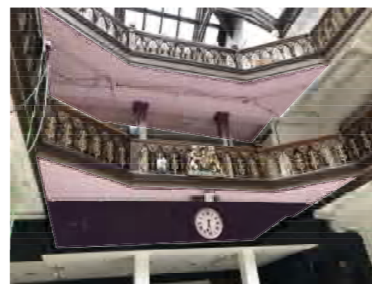
NORTH END OF ATRIUM (FROM GROUND FLOOR)
