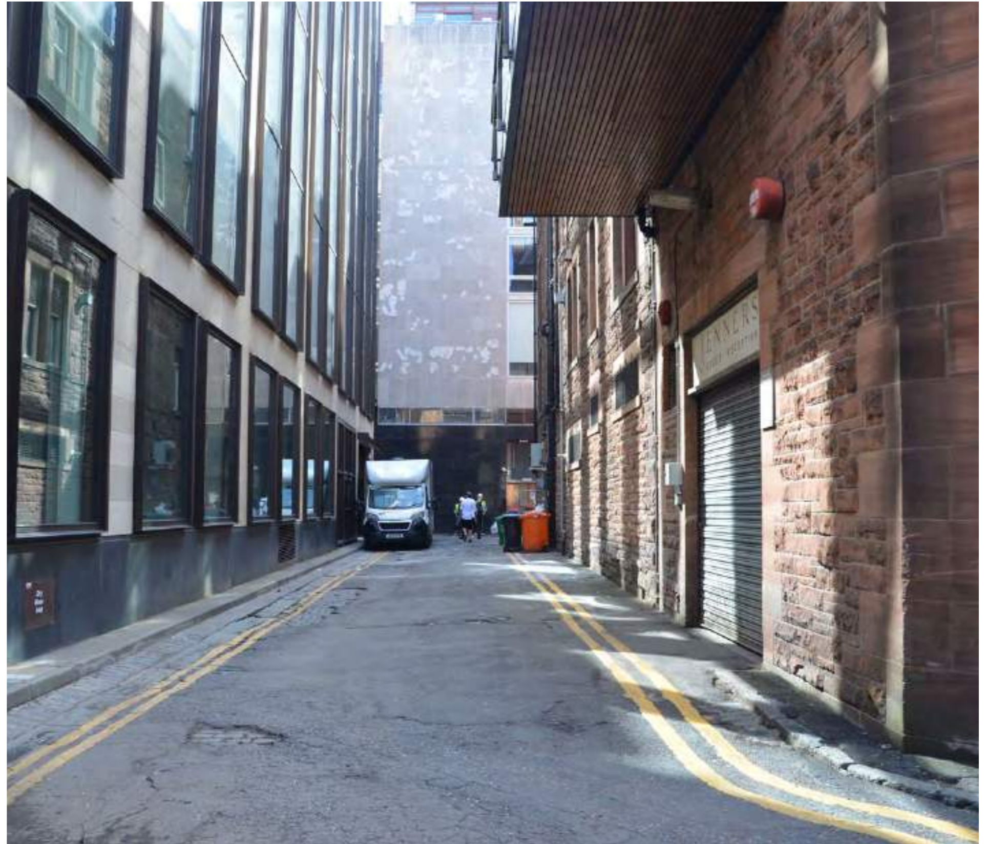
Rose Street North Lane service bay behind Abbotsford Building
