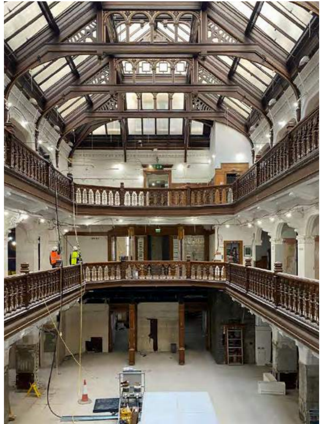
Existing atrium photograph
