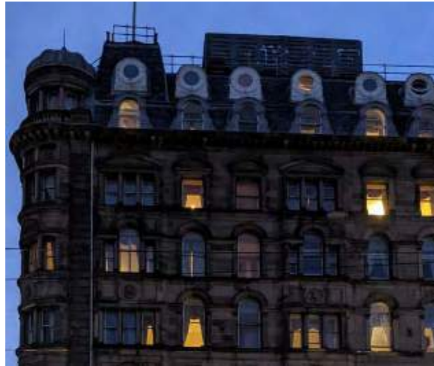
Occupancy lighting determines night time identity. It is key to consider the different uses and extents in elevation, from open plan retail areas, to individual hotel bedrooms.
