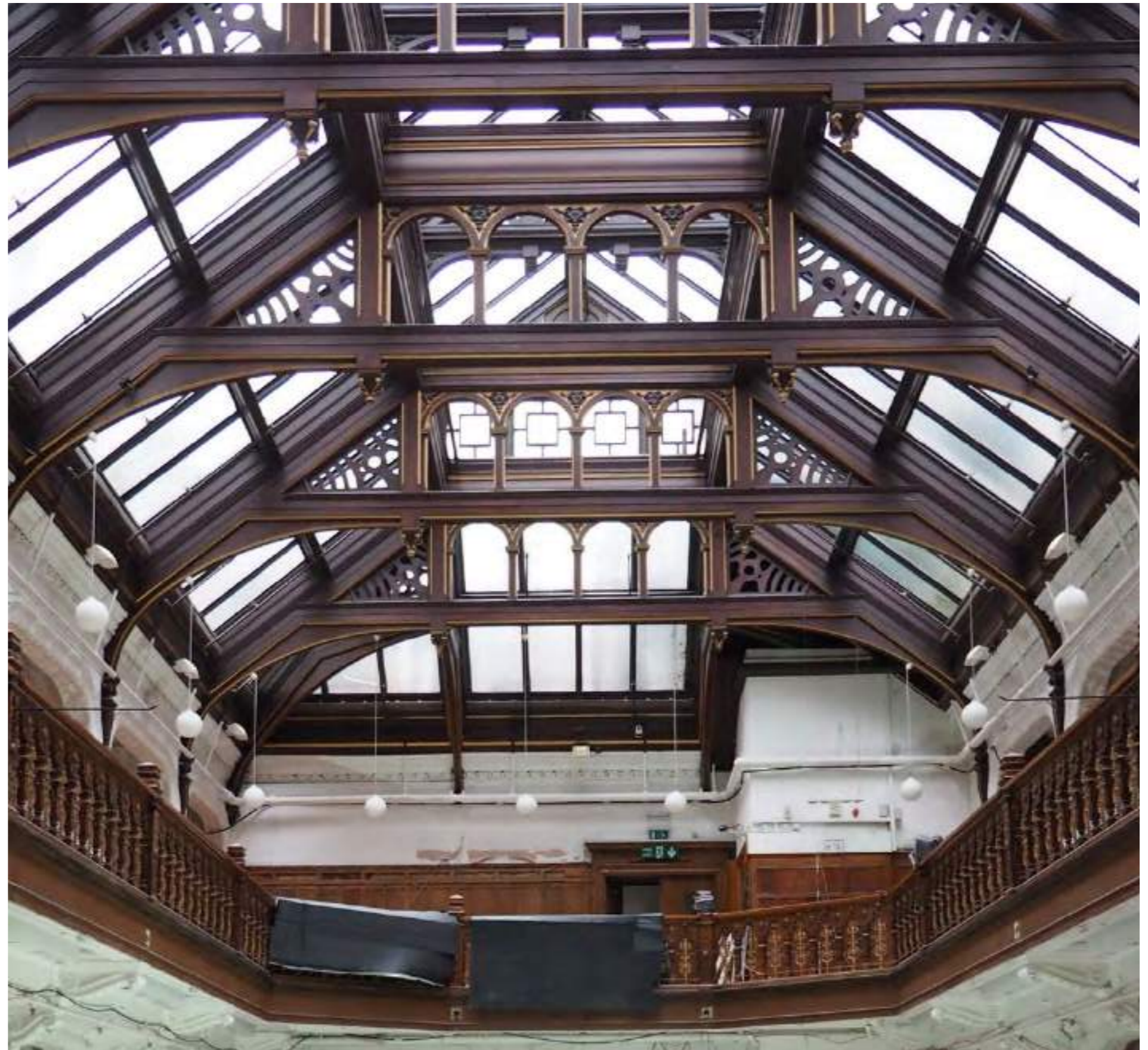
Current condition of atrium roof
