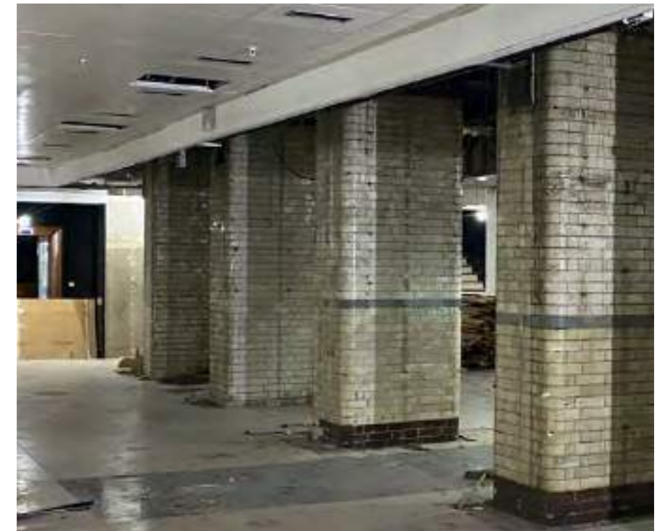
Glazed brick features throughout in the basement and back of house areas
