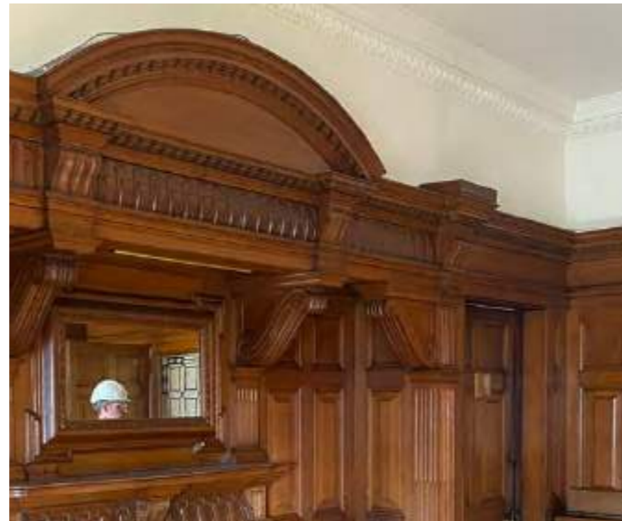
Third floor board room timber wall panelling
