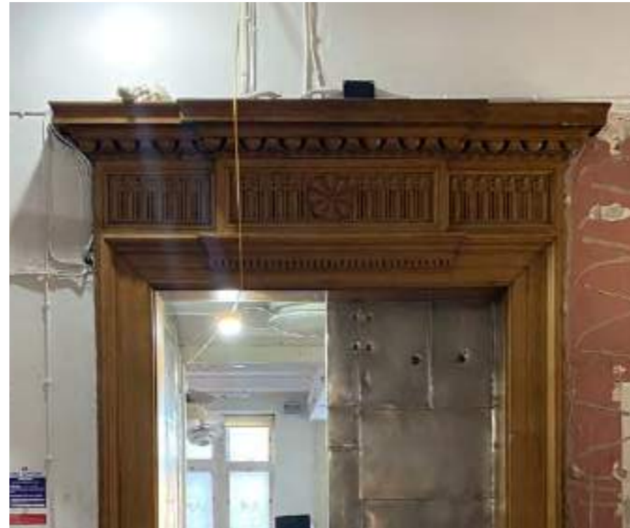
Timber door thresholds are a consistent feature throughout
