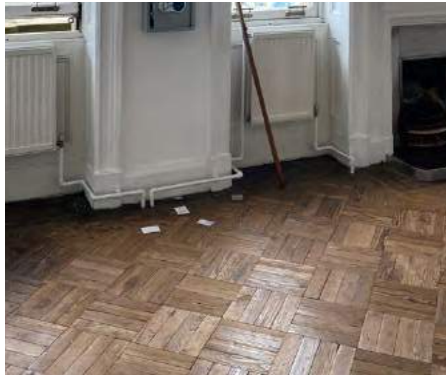
Original parquet flooring on third floor
