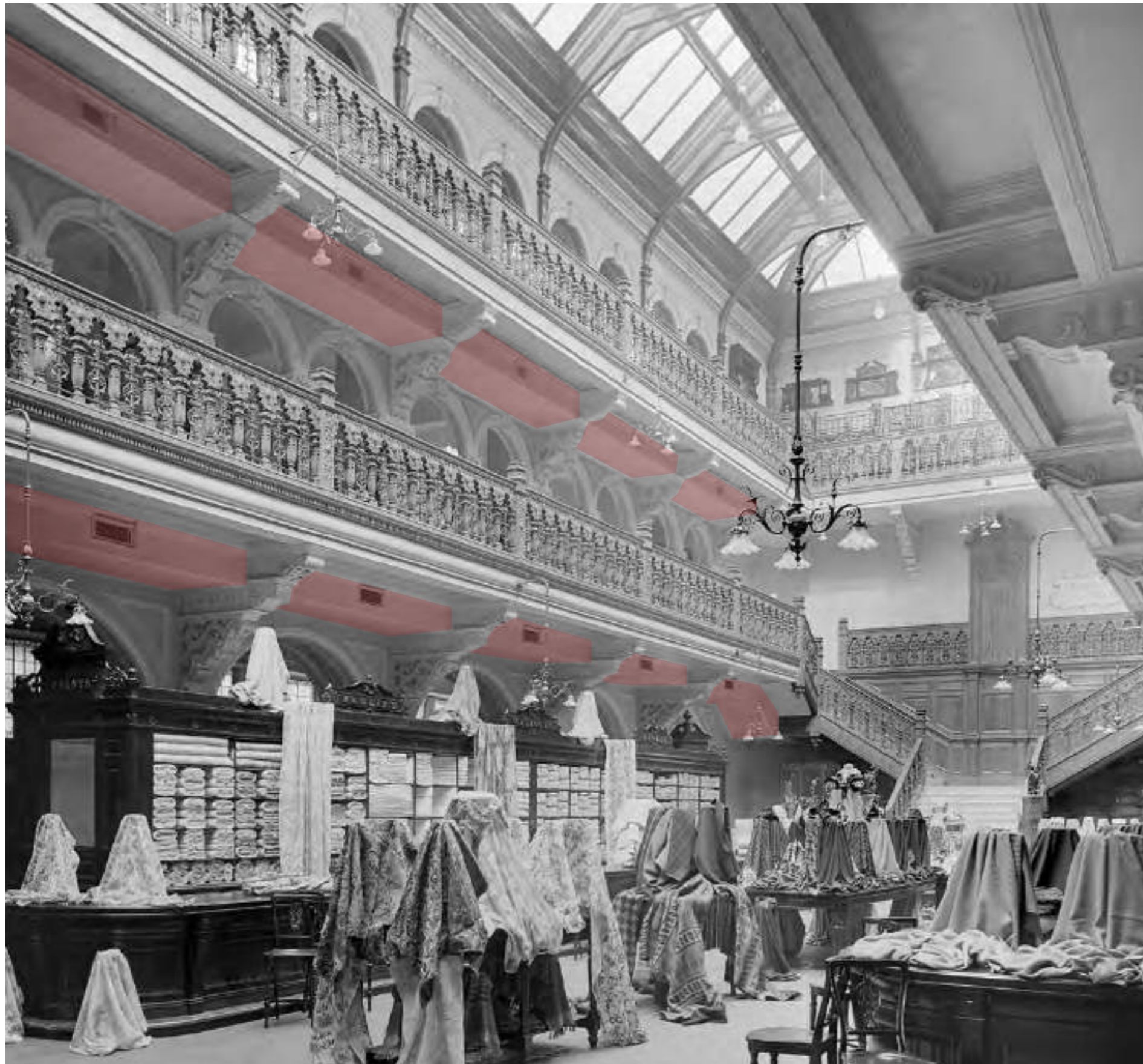
Ventilation was integrated into the original design of the atrium
