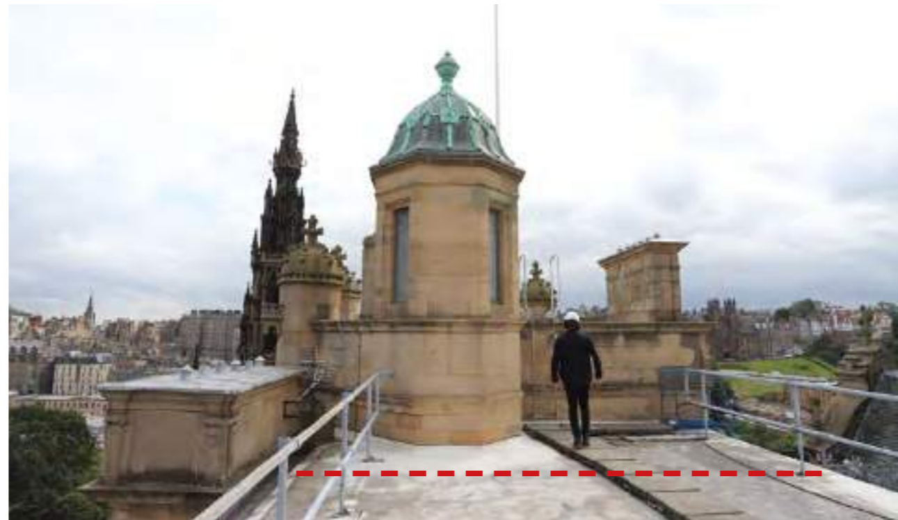
Princes Street corner tower photograph from site visit August 2021 - dashed red line indicates proposed 7th floor roof edge
